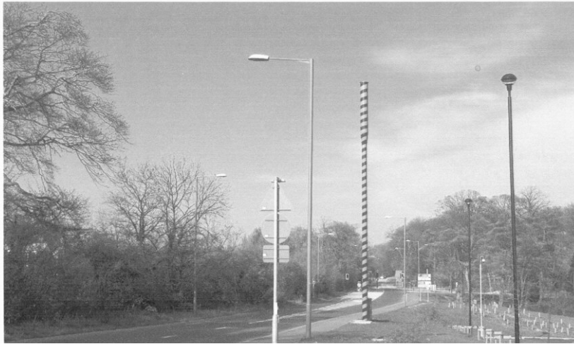
O2 monopole, South Road (D. Jones)
