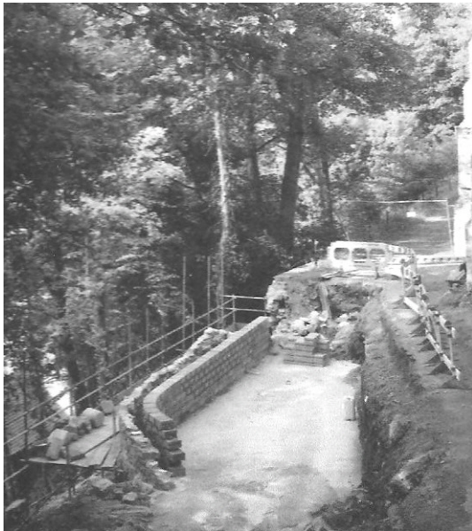
High-level Riverbank under repair. (D.Pocock) Association of British Market Authorities.
