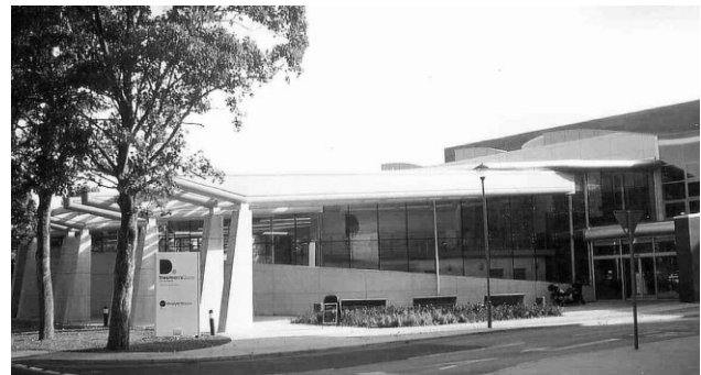
Leisure Centre from Freeman's Place (Photo: D. Pocock)
